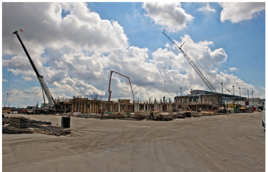
Pumping Jet Wall Gate Towers
