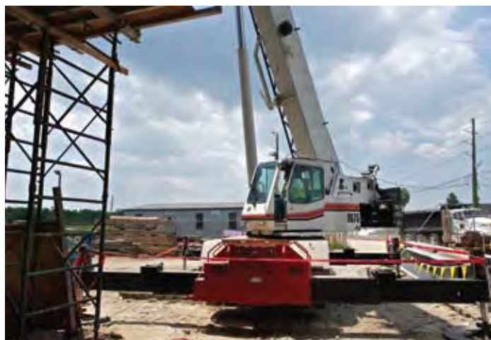
75 ton concrete crane in action
