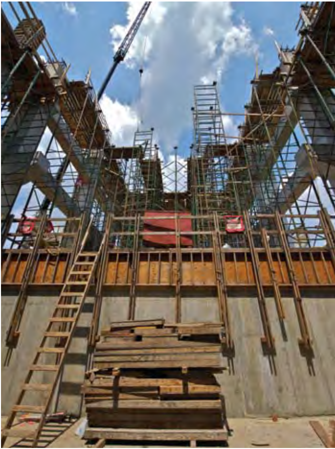
New generator building
