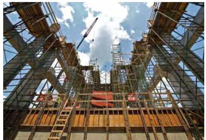
New generator building
