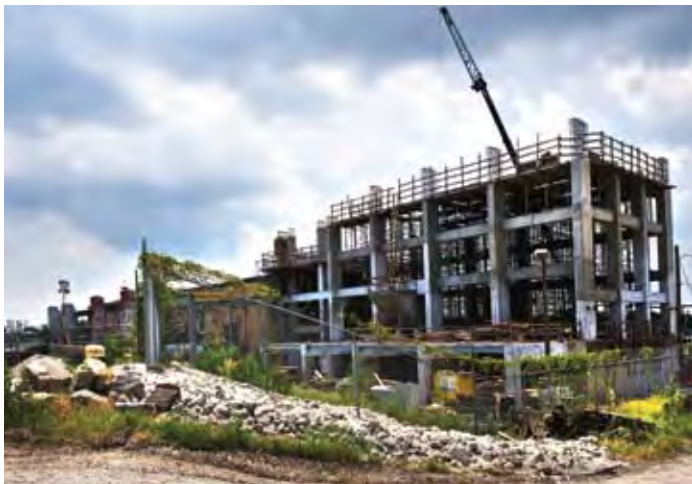
East elevation of new generator building
