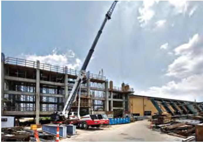
West elevation of existing pump station and new generator building
