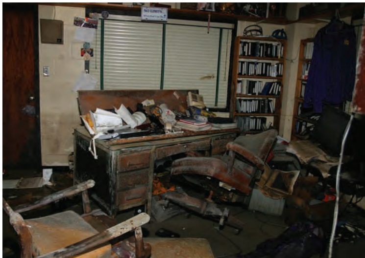
With a $1 million cleanup cost, restoration of St. Augustine High School included removing damaged sheet rock, mold, and wet flooring.
