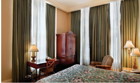
Construction took place in every room, some of which had to be completely gutted to clear out debris and mold.
