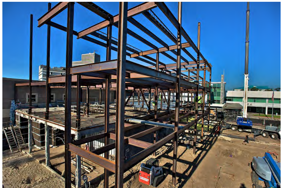
Structure Taking Shape
