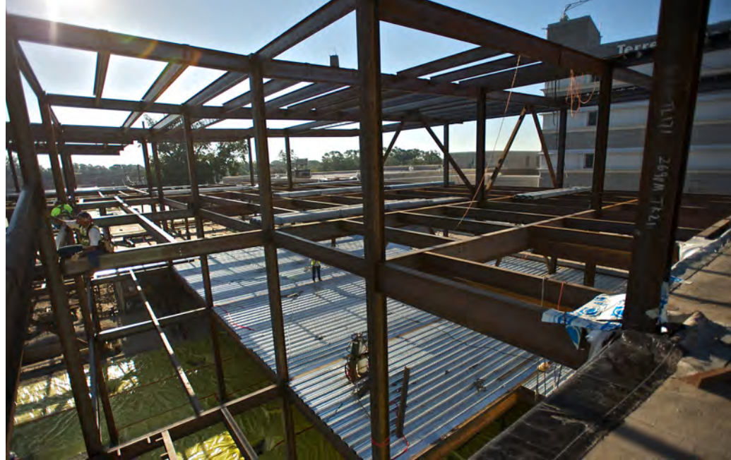
Steel and Decking Work Moves Project Forward
