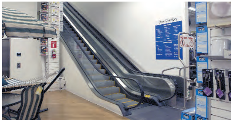
The cart carrier and escalator are side-by-side providing customers the convenience of transporting their shopping carts to the second floor via escalator.
